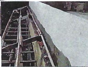
REPAIRS TO EAVES
