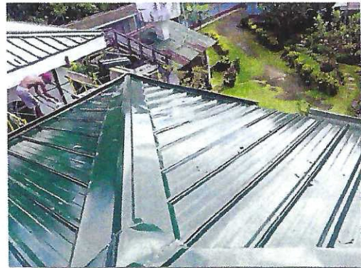
MAGNIFICAT BUILDING'S NEW STEEL ROOF
