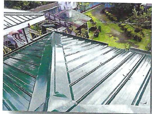
MAGNIFICAT BUILDING'S NEW STEEL ROOF
