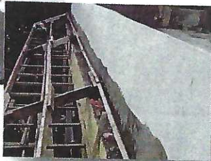
REPAIRS TO EAVES
